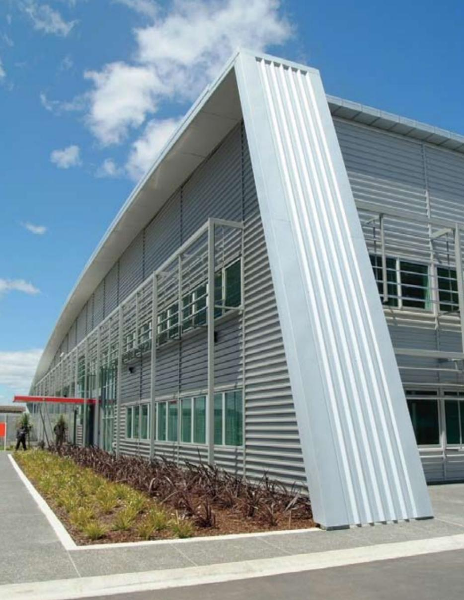
Prominent acrylic panels at the entrances outline the building's sustainable features, which include unpainted Zinalume® cladding for the roof and Colorcote® ZR8™ wall cladding.
