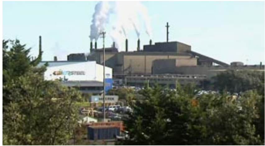
The New Zealand Steel Mill, Glenbrook, Franklin, New Zealand.
