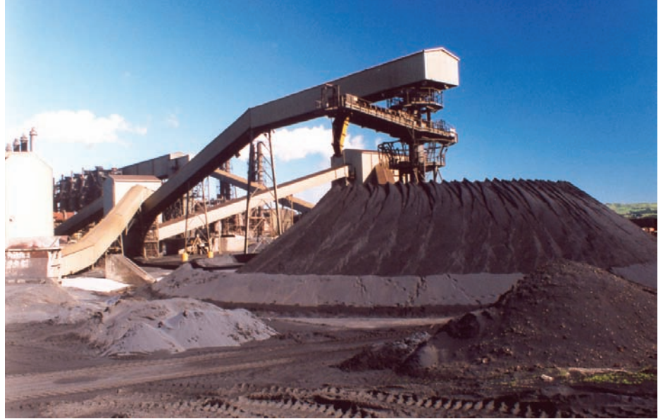
Iron sand is concentrated using double drum magnetic separators and further cleaned before stock piling.
